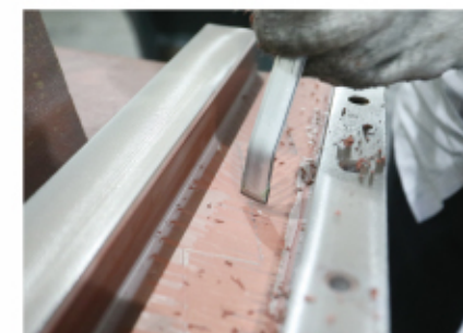
Scraping of Joint Surface
